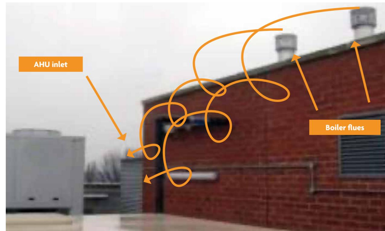
▲ **Figure 4. Discharges from boiler flues at low height ingressing into the building AHU.<sup>19</sup> (© BRE)**
