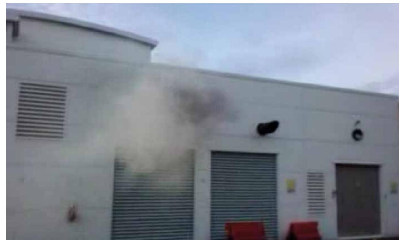
▲ **Figure 5. Emissions from a hospital's back-up diesel generator discharging horizontally.<sup>19</sup> (Low-resolution screenshot of video footage; © BRE)**
