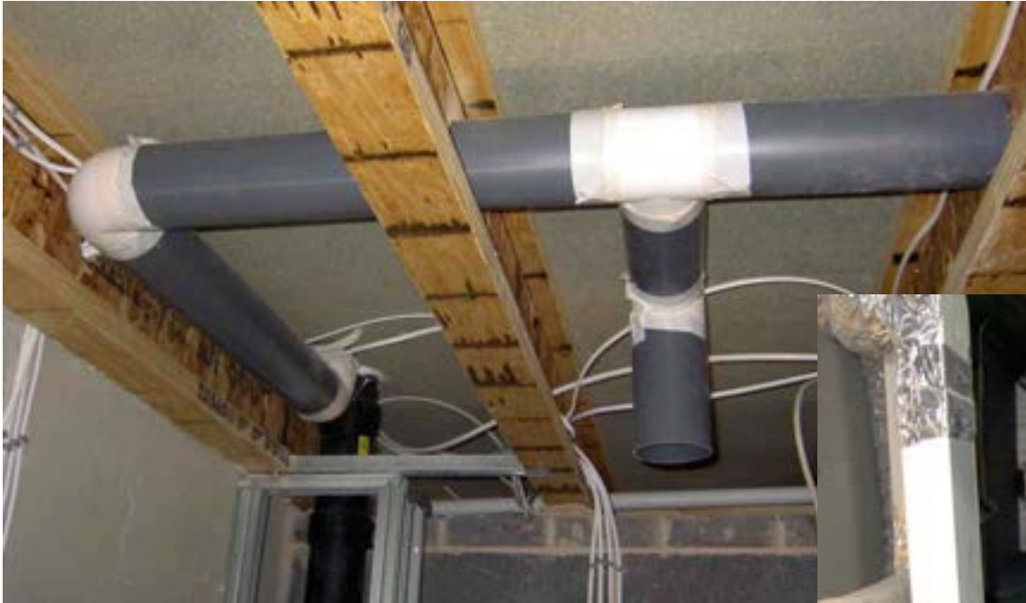
Duct mechanically fixed and silicon sealed
